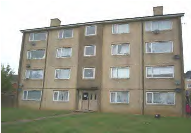
Photograph 23: Lewes House, Front Elevation.
