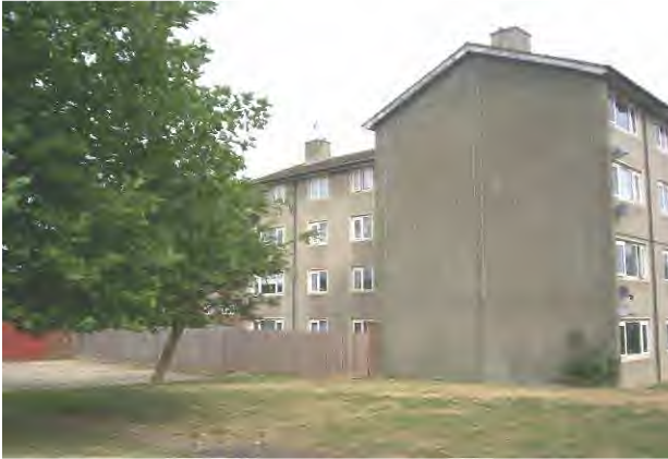
Photograph 18: Fife House, Left Hand Gable Elevation.
