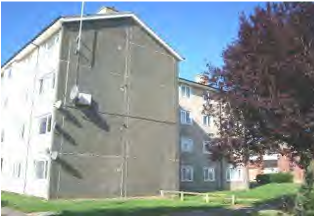
Photograph 28: Pembroke House, Right Hand Gable Elevation.
