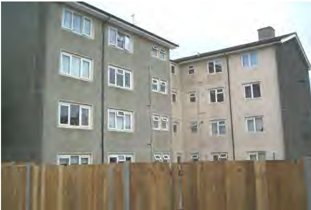
Photograph 31: Rutland House, Left Hand Gable Elevation.
