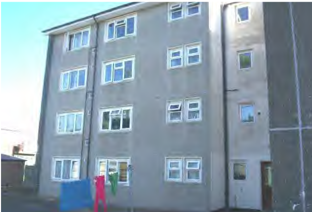
Photograph 27: Pembroke House, Left Hand Gable Elevation.
