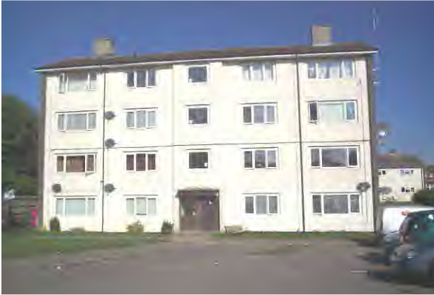
Photograph 26: Pembroke House, Front Elevation.
