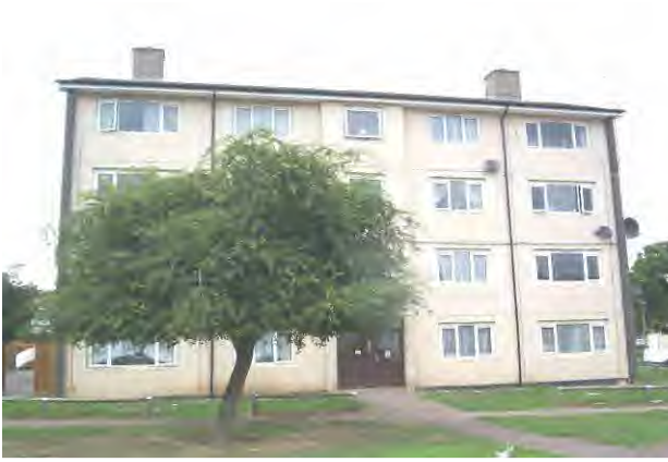
Photograph 29: Rutland House, Front Elevation.
