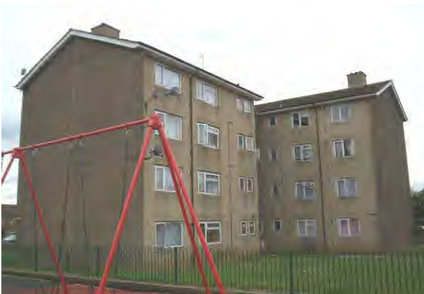
Photograph 24: Lewes House, Left Hand Gable Elevation.
