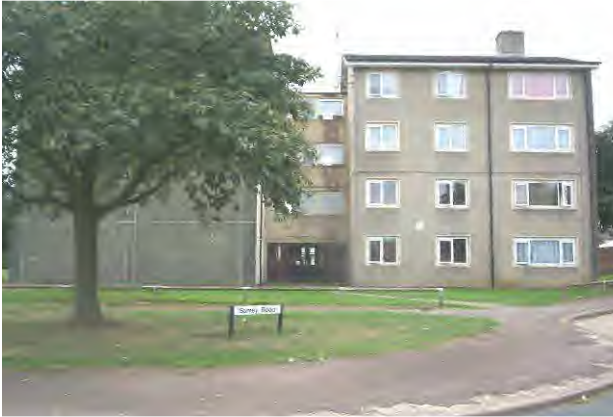
Photograph 30: Rutland House, Right Hand Gable Elevation.
