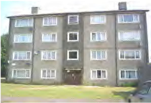
Photograph 1: Norfolk House, Front Elevation.
