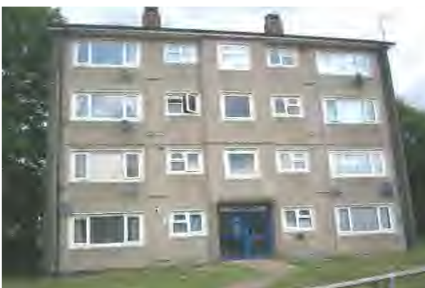
Photograph 4: Sawley House, Front Elevation.
