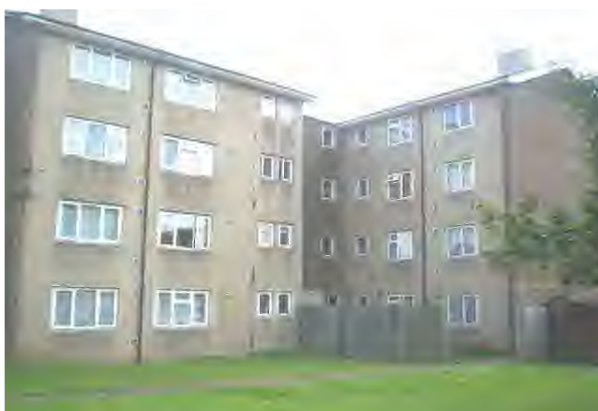
Photograph 8: Stirling House, LH Gable Elevation.
