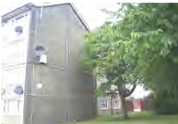
Photograph 6: Sawley House, RH Gable Elevation.
