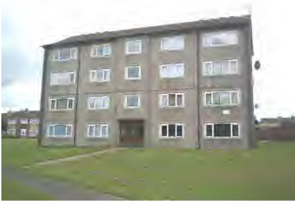
Photograph 10: Waltham House, Front Elevation.
