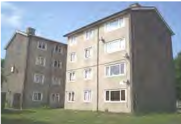
Photograph 3: Norfolk House, RH Gable Elevation.
