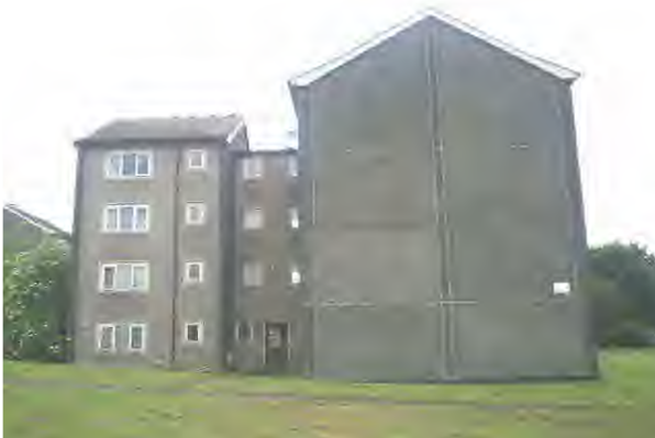
Photograph 11: Waltham House, LH Gable Elevation.
