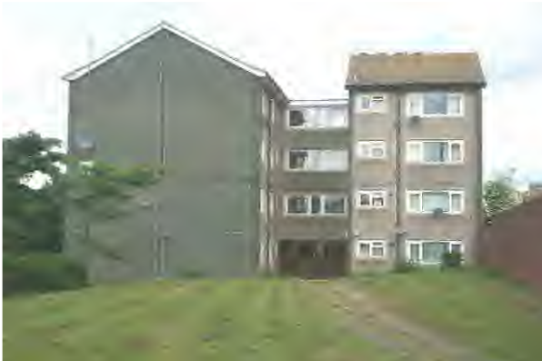
Photograph 12: Waltham House, RH Gable Elevation.
